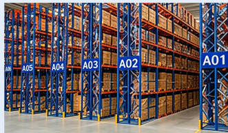
Storage Racking Systems
